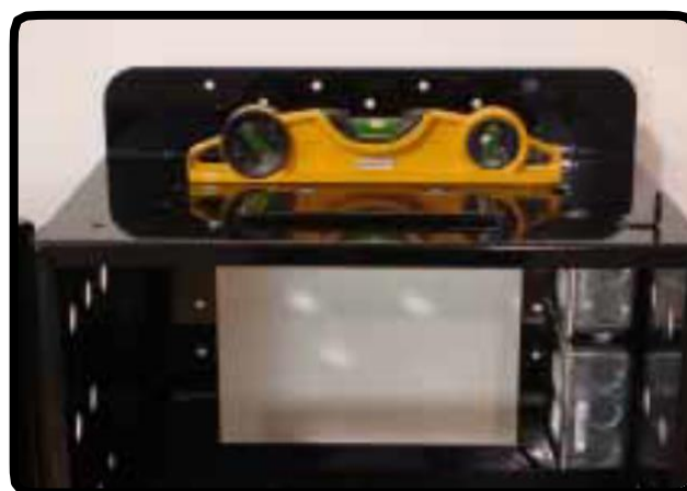
Level and place the second screw.
