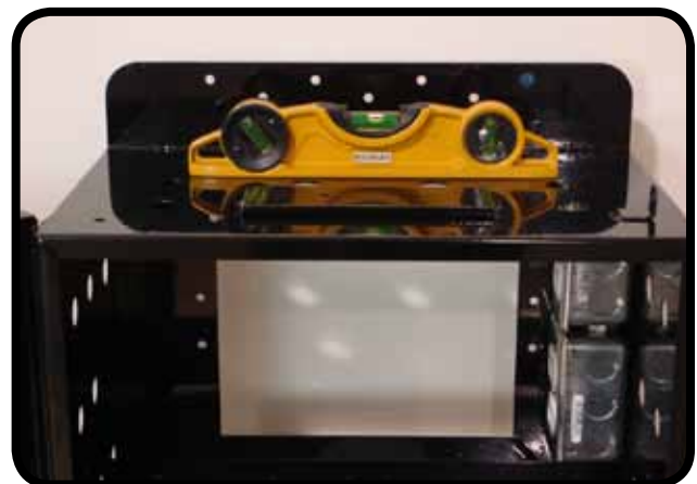
Level and place the second screw.
